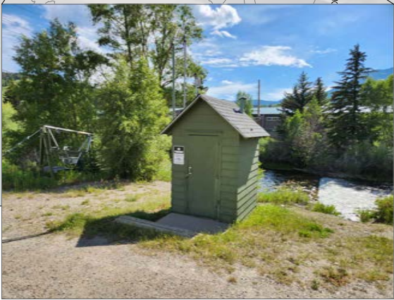
EXISTING USGS STREAM GAGING STATION
